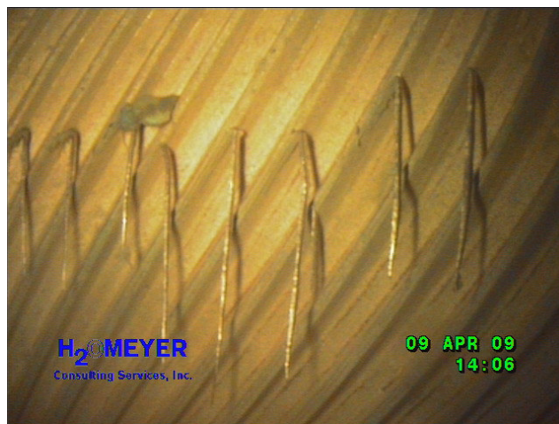
Row 30, Tube 41 – Manufacture defects of tube enhancements.
